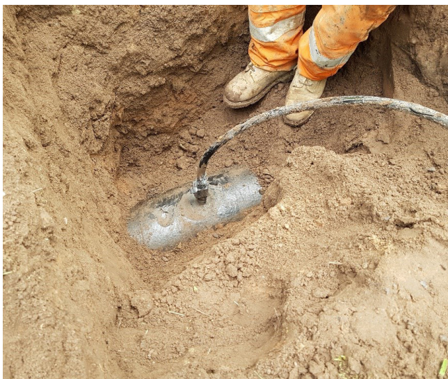
Figure 6. A tapping point exposed by the pipeline operator.
