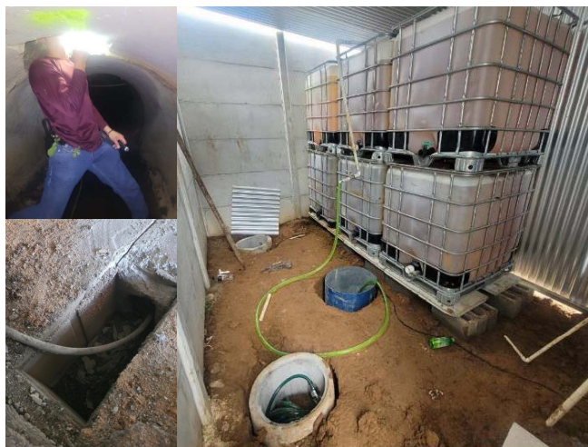
Figure 4. The tunnel used by thieves in Costa Rica (top left) for their tapping point route (bottom left) which led to storage containers at a private property 300 m from the tapping point (right).
